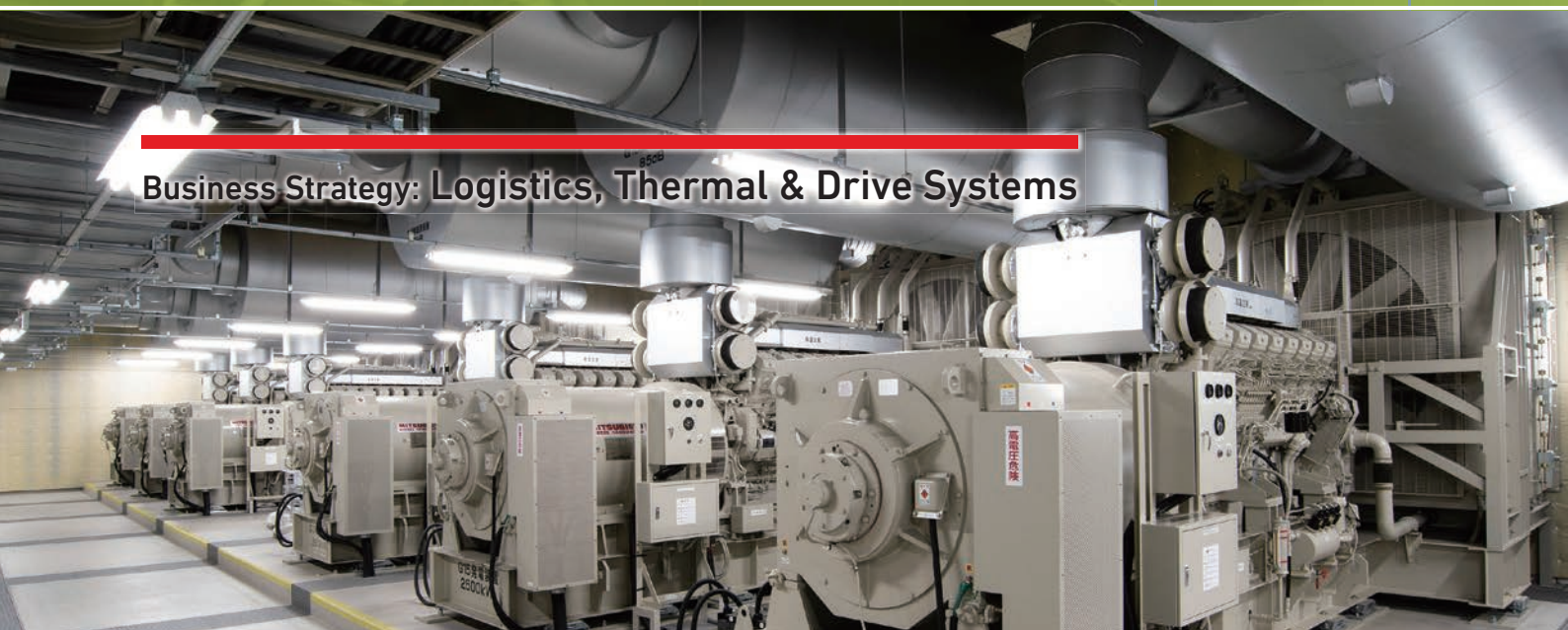
Engine Generator Sets for Data Centers
